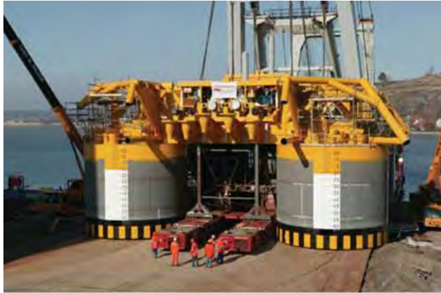
It took the world's largest crane barge to lower an Ormen Lange template to the sea floor. (Photo by Mediafota as, courtesy of FMC)
