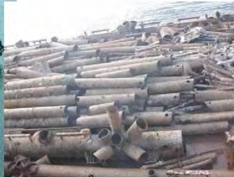
Decommissioned in Pieces (Major subsea cutting needed)
